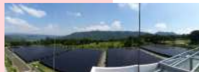
Gambar 3. 5 Array 31 (Ground Mounted)
