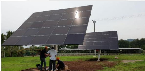
Gambar 2. 1 Single axis solar tracker
