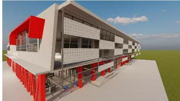
Gambar 11 Sun shading
