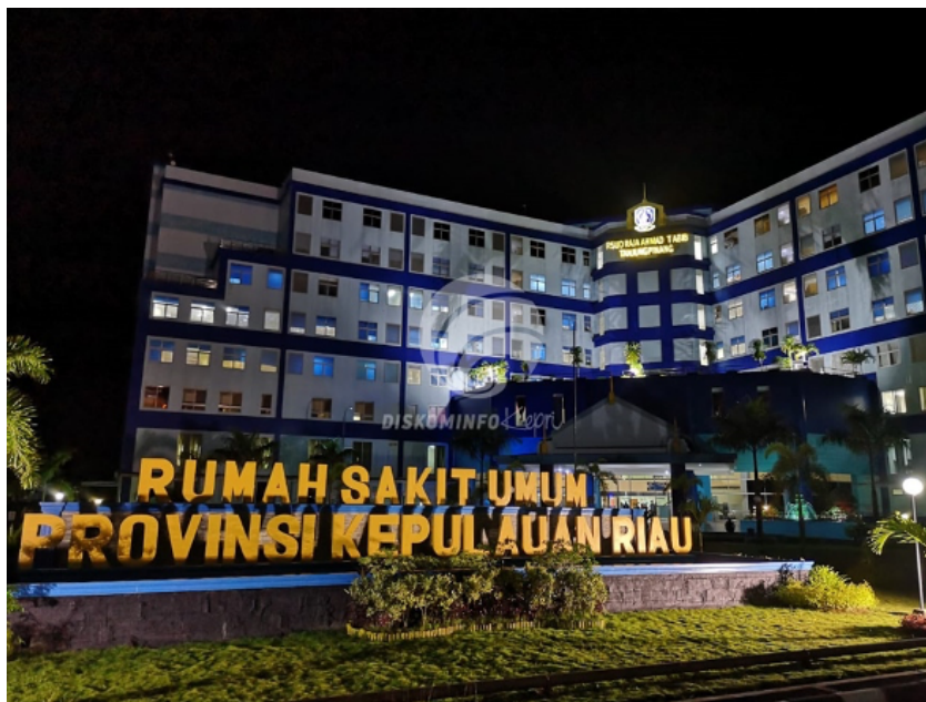
Figure 1. 1 Image of Raja Ahmad Tabib Provincial General Hospital
