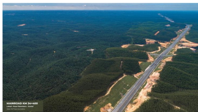
Gambar 1. 3 Mainroad Ruas Tol Pekanbaru Dumai
