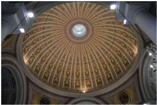
Fig. 8. Internal view of the dome.
