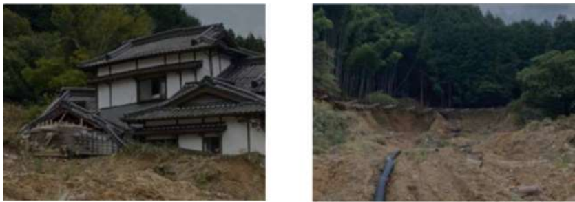
Fig. 4. Landslide field in Soeda-Cho, Japan
