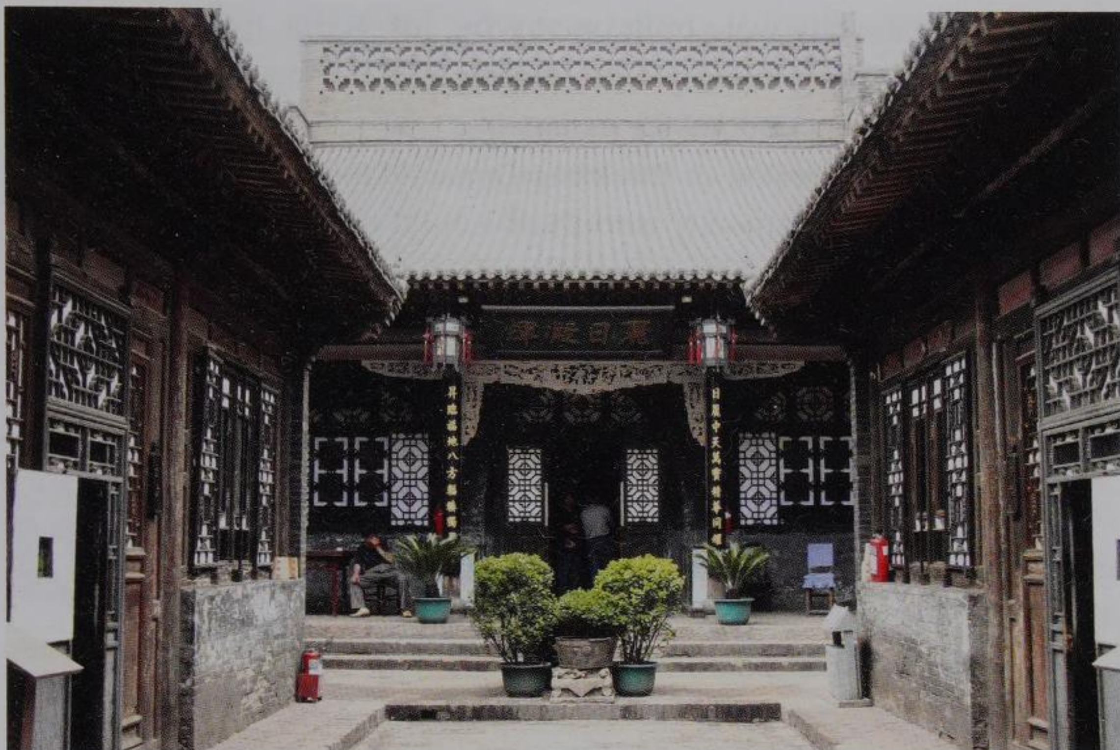
Inner yard of the Rishengchang draft bank, Pingyao, Shanxi Province.
