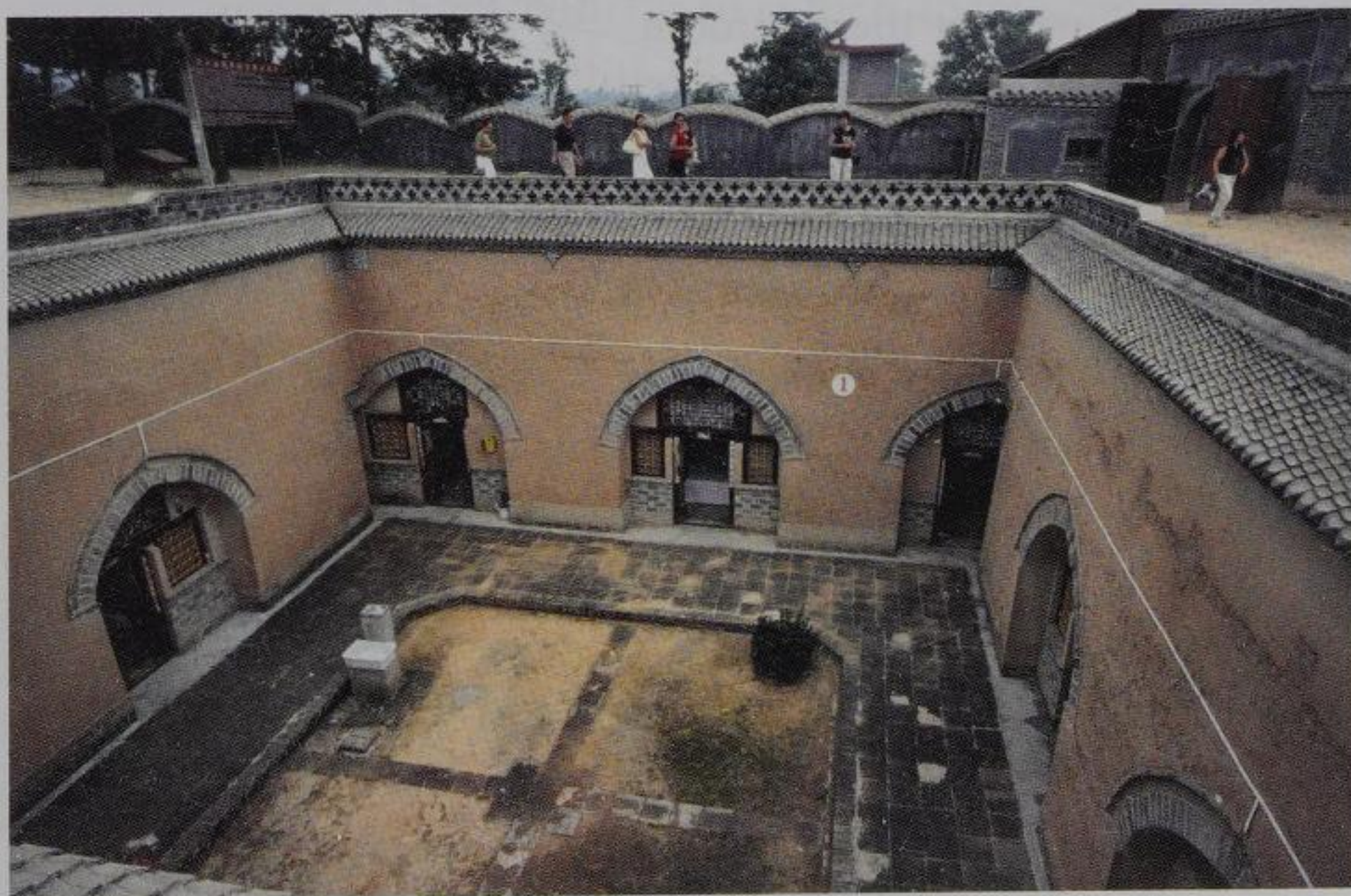
Courtyard cave dwellings, Shanxian County, Henan Province.
