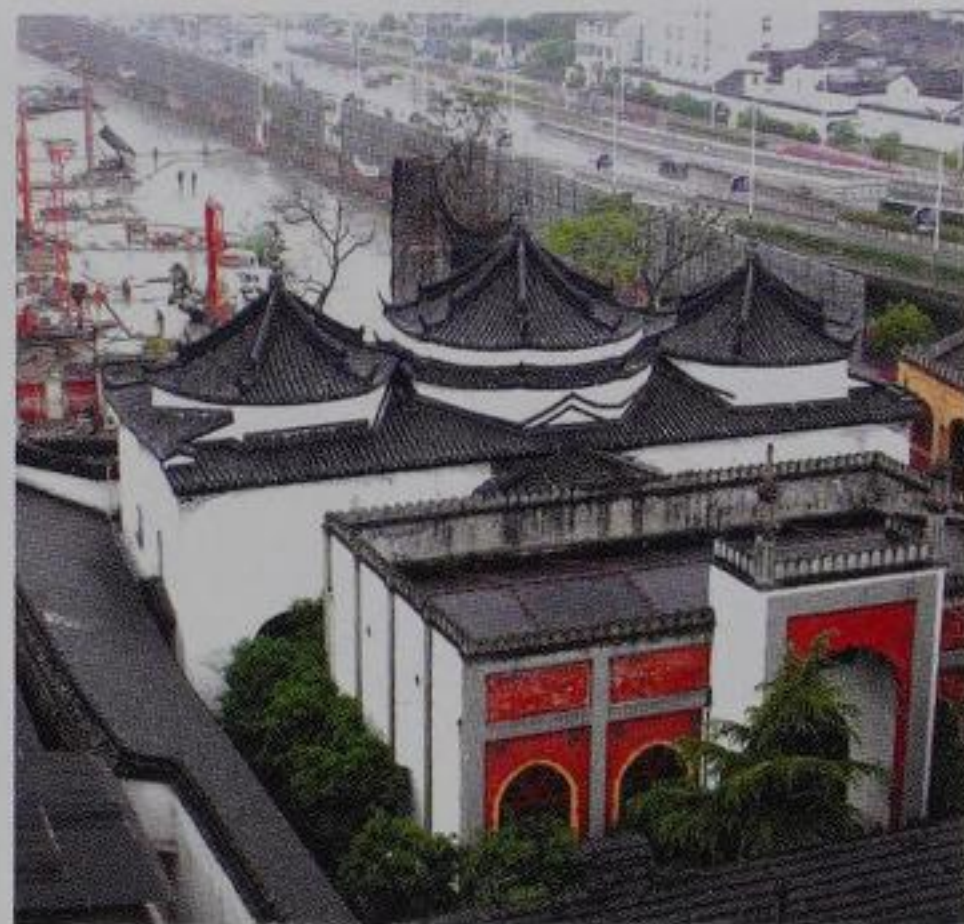
The roof of Fenghuang Temple (Phoenix Temple) in Hangzhou displays a blend of the traditional Chinese and Islamic architectural styles.
