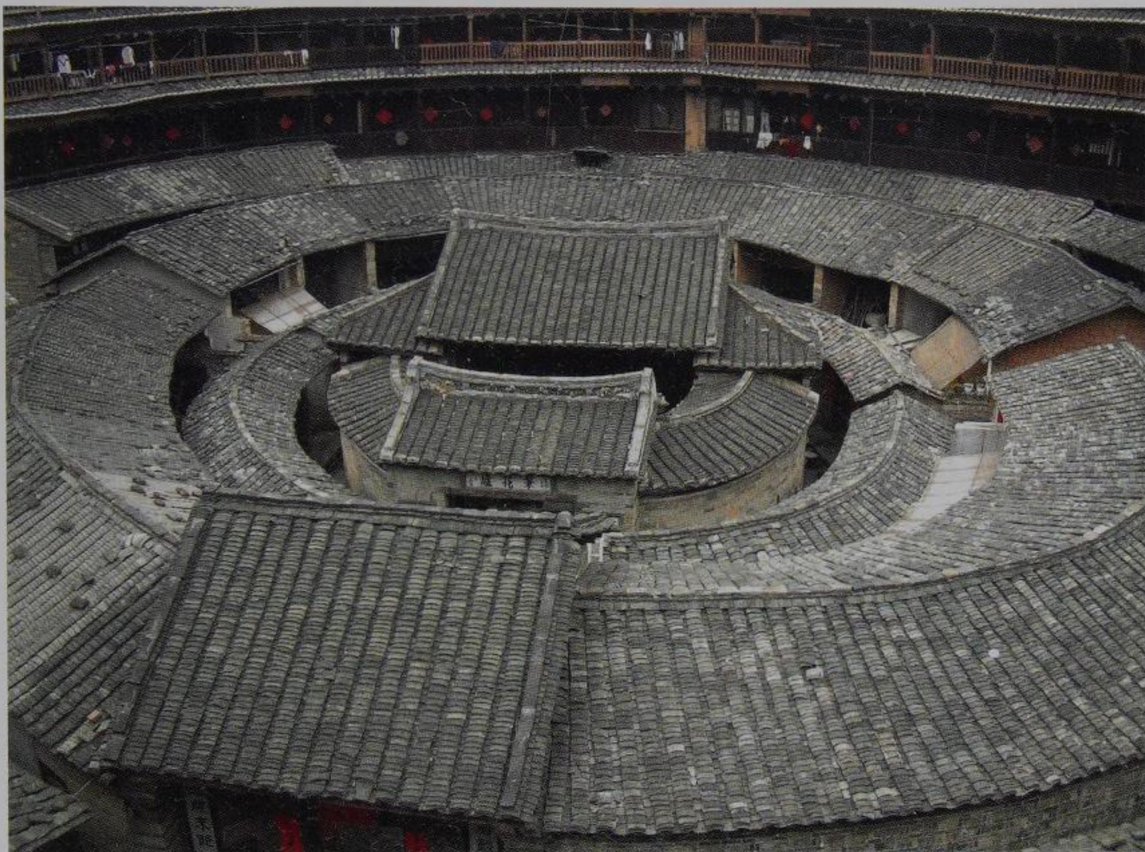
The inner ring of Chengqi House, Yongding, Fujian.
