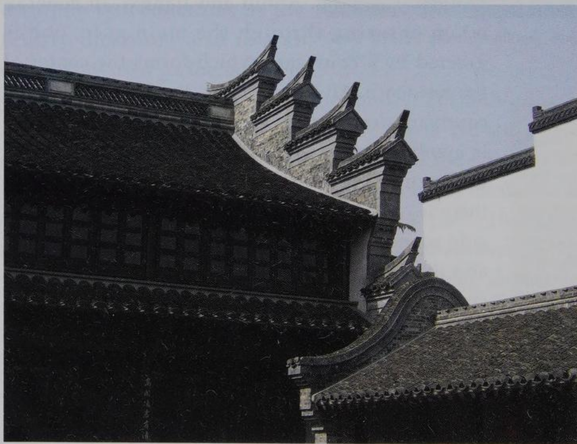
White, cascading small roofs forming a "Horsehead Wall".
