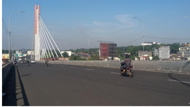
Figure 4. 7 Jalan Layang Pasopati (Source: Private Document, 2024)
