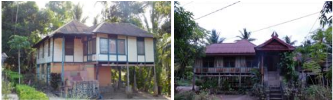
Figure 10. Bugis noble house build in 1960's Andi Abidah, 2015
